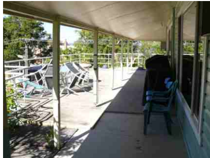
Verandah outside main kitchen dining area with BBQ
