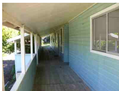
Verandah outside flats 1 & 2
